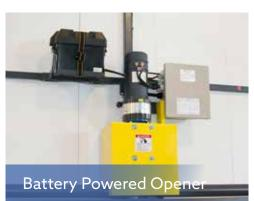
Doors can be equipped with a battery powered DC opener, ideal for remote locations where line power is not available.
